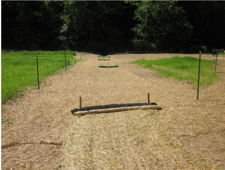
*A wide variety of sediment and erosion control materials and products are available to minimize the effects of precipitation before vegetation can be established.*
