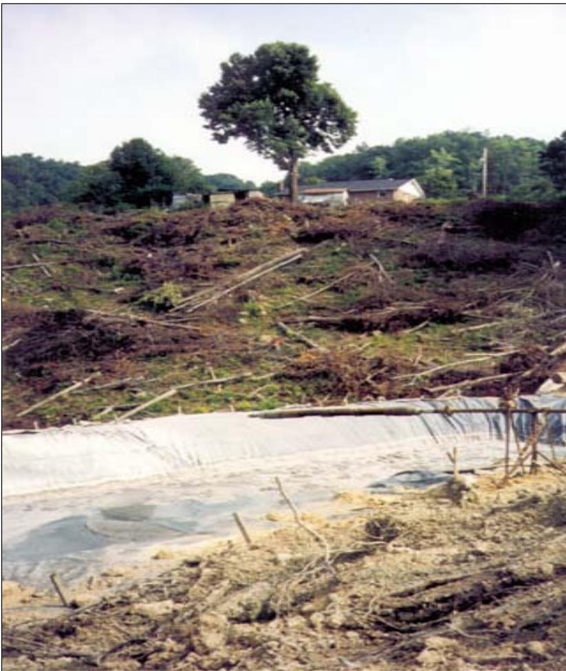
Figures 4-10 and 4-11. Fluid that is extracted from the well is sprayed through a diffuser and stored in a lined trench until it is disposed of off-site or discharged.
