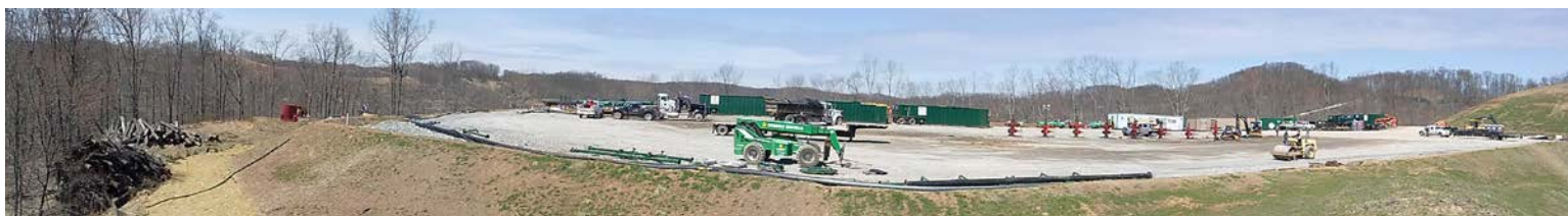
Photo taken after drilling but before completion that contrasts EQT's Marcellus Shale well pad with the site of a vertical well drilled in 1995 immediately next to it, at left. This site is subject to a surface use trespass case. See details below.
