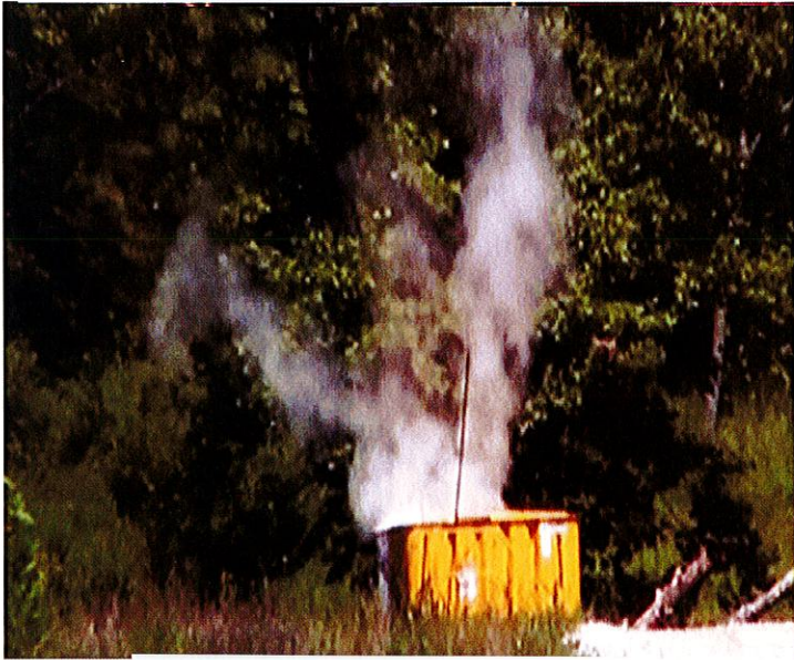
Pipeline Condensate Tank
