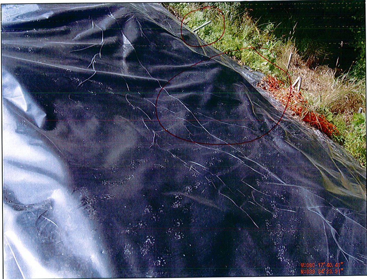
Figure 11: Downstream Slope Movement into Ditch
