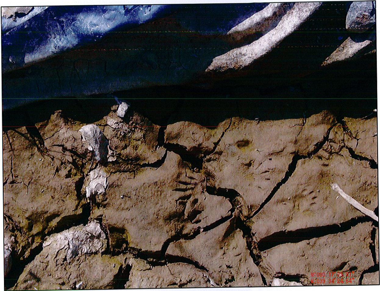
Figure 4: Settlement Cracks in Anchor Trench
