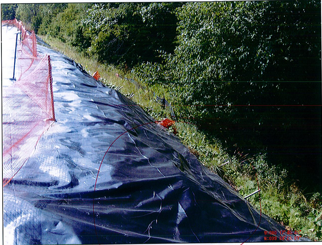
Figure 5: Bulges on Downstream Face
