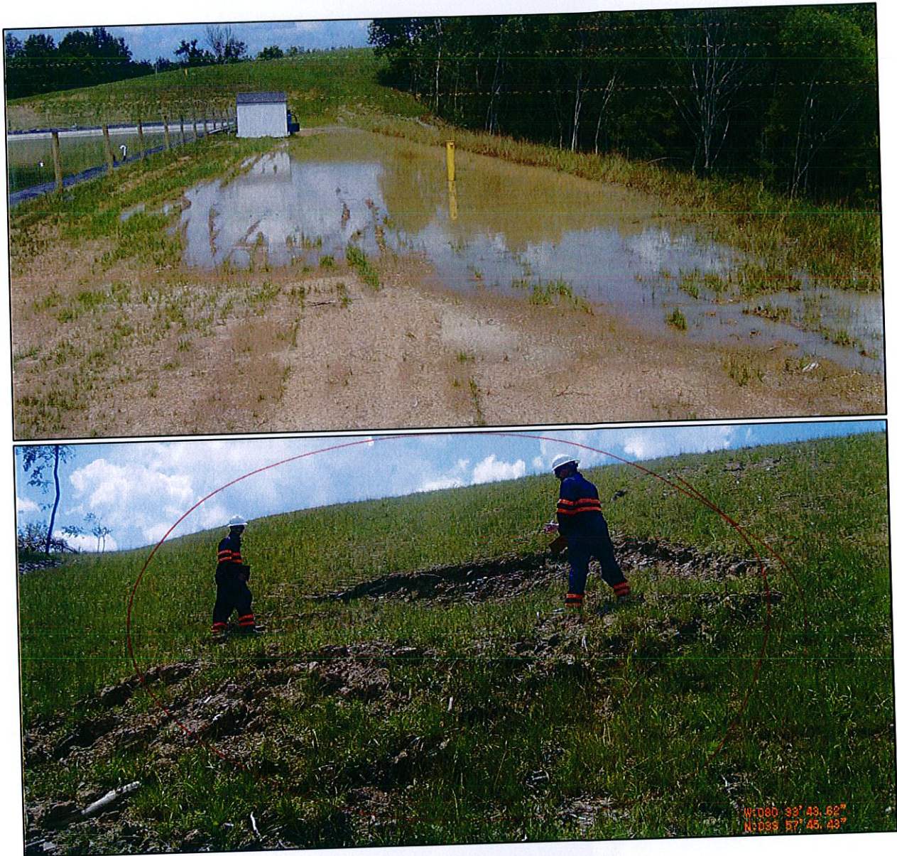
Figure 13: Slope Movement at SHL 4
