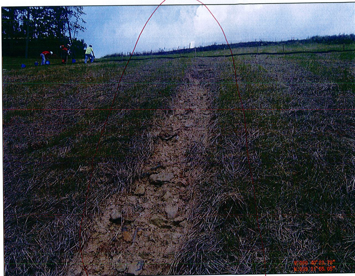
Figure 12: Surface Erosion at Mills-Wetzel
