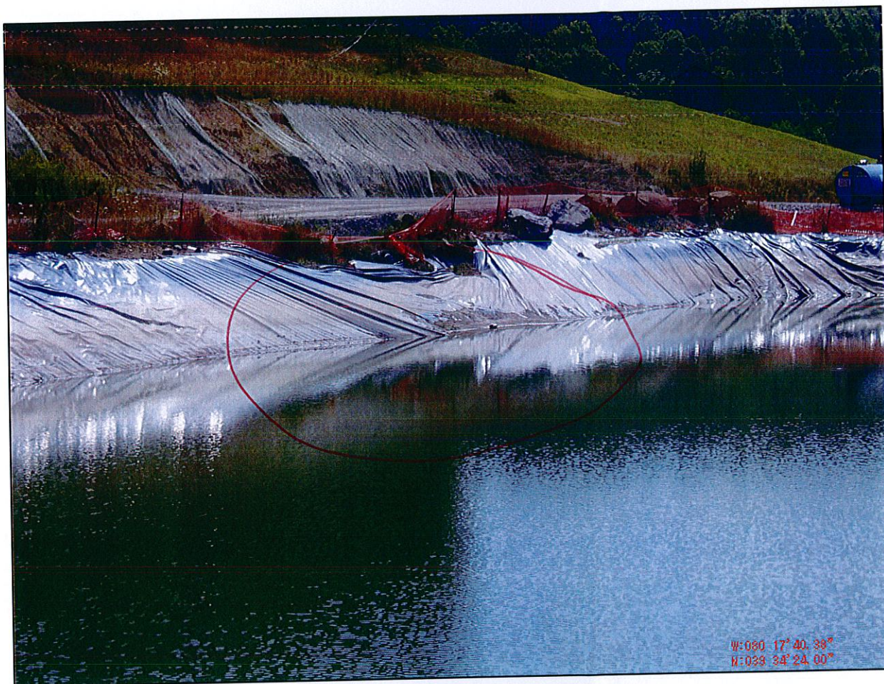
Figure 6: Slope Movement into Impoundment
