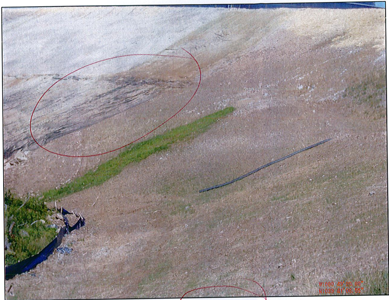
Figure 15: Seepage at Pribble
