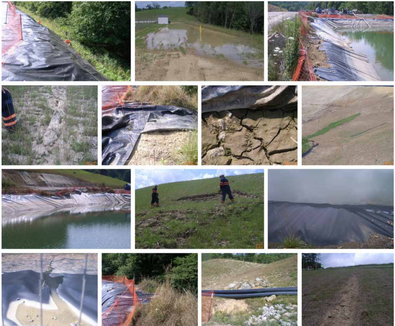
Documented problems with pit identified during a study conducted by WVU. (Source: Pits and Impoundments Final Report Assessing Environmental Impacts of Horizontal Well Drilling Operations , WVU Department of Civil and Environmental Engineering, December 17, 2012.)
