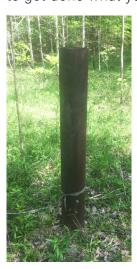
This is what a well should look like after it has been plugged. If there is more there than this required "monument" of the plugged well, then it has not been plugged and it is either producing or should be plugged. Look up its production/status using the "API" number that should be on it (should look like 047-0??-0????). For more info on API numbers & uses, go to "More Helpful Links and How To Find Information on Particular Gas Wells" on our website.
